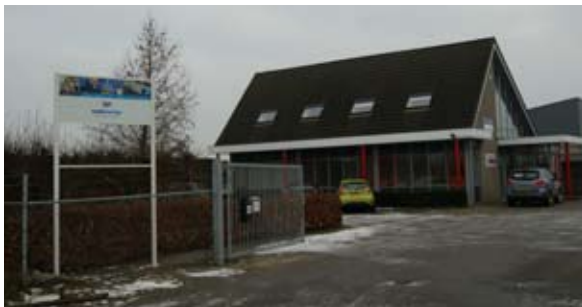
Cool Energy's New Depot
