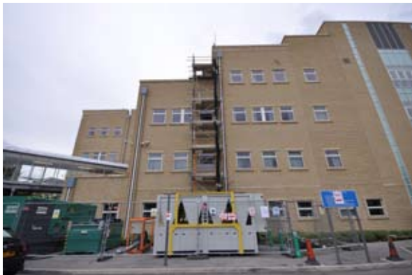
The customers building with chillers sited externally
