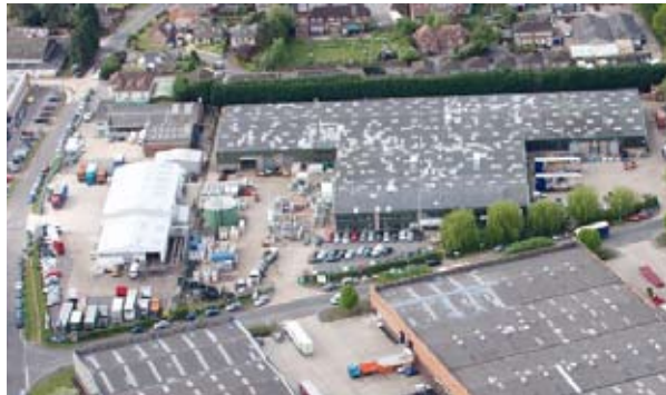
The Cool Energy Head Office, Totton, Southampton.
