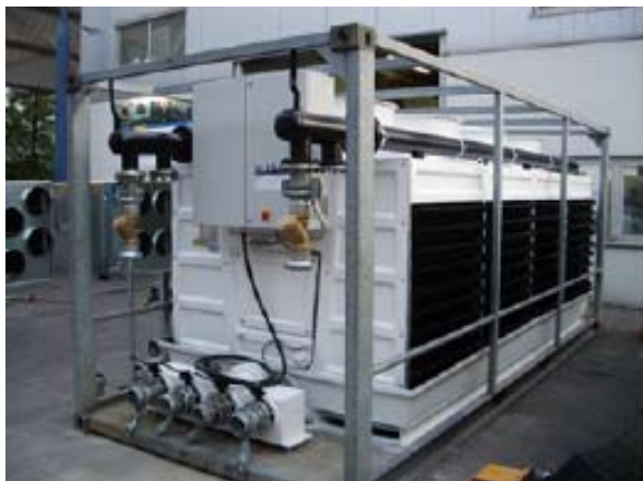
Cool Energy 2.5mW Rental Cooling Tower
