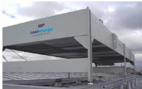
Cool Energy 500kW Rental Air Blast Cooler
