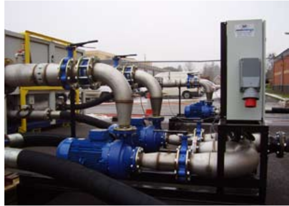
The Pumping Station
