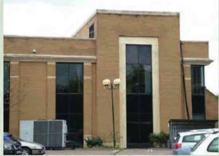
Low noise equipment cooling a data storage facility
