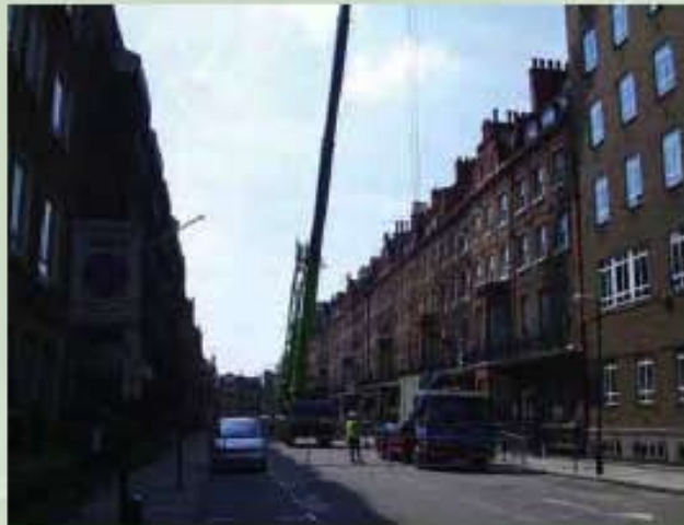
Cool Energy managing lifting, road closure and project installation
