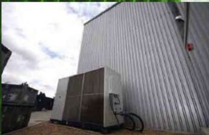
150kW cooling package with small footprint
