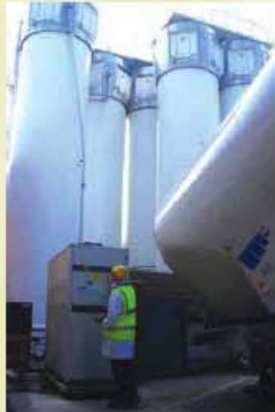
Cooling a biscuit production line
