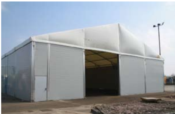
The Installed Chill Store
