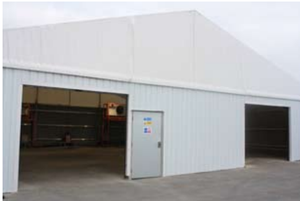
The Installed Chill Store
