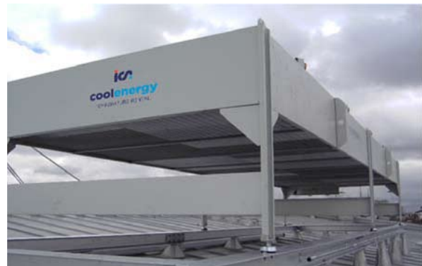
Cool Energy 500kW Rental Air Blast Cooler
