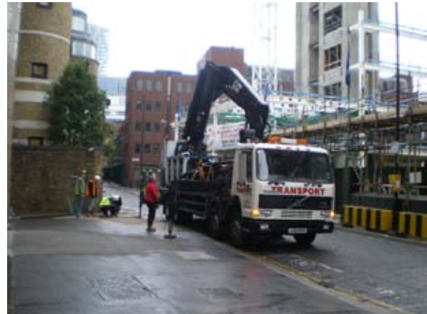
Cool Energy sub-contract a local lift and shift company
