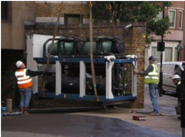
Cool Energy engineers install the water-cooled chiller
